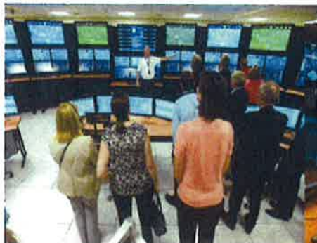
The NuScale Power simulator control room design brings together decades of Digital I&C, Human Factors Engineering and Human Systems Interface research and field experience.
