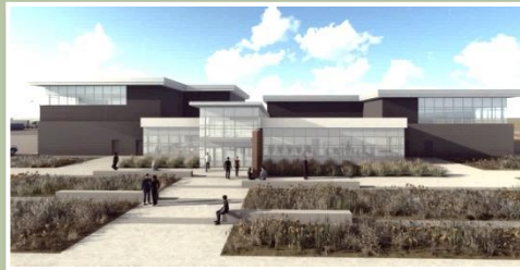
Maintenance Support Building
