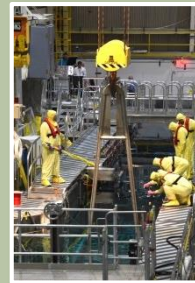
30-Ton and 40-Ton Crane Replacements
