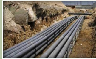
Utility Corridor Modernization
