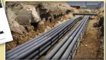
Utility Corridor Modernization
