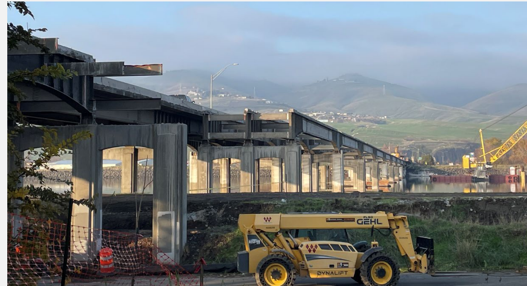
US-12 Clearwater Memorial Bridge, Lewiston
