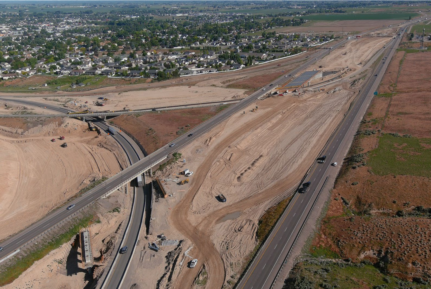
I-86/I-15 System Interchange Reconstruction, Pocatello
