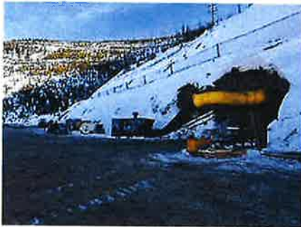
Portal Bench infrastructure supporting underground activities
