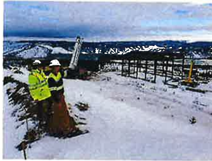
Surface facilities overview
