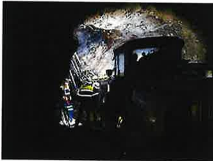
Progressing underground development works
