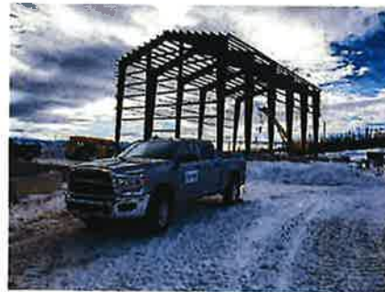
Flotation building progress
