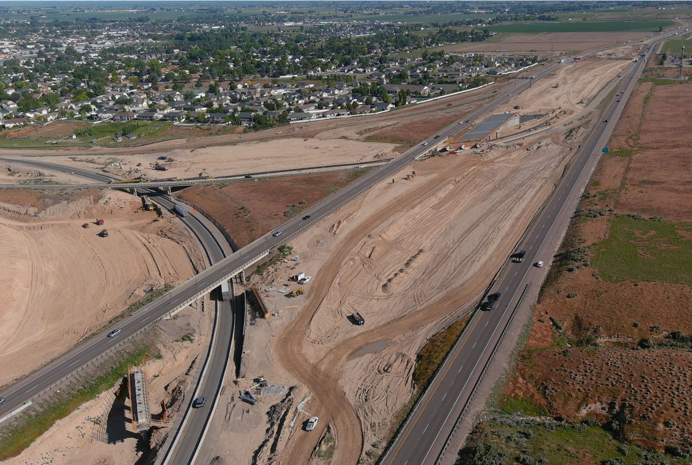
I-86/I-15 System Interchange Reconstruction, Pocatello
