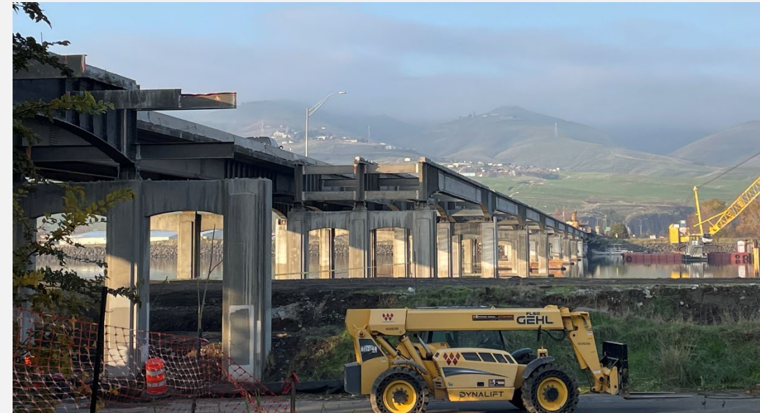
US-12 Clearwater Memorial Bridge, Lewiston
