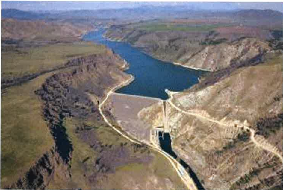
Anderson Ranch Dam and Reservoir – Planned for Enlargement
