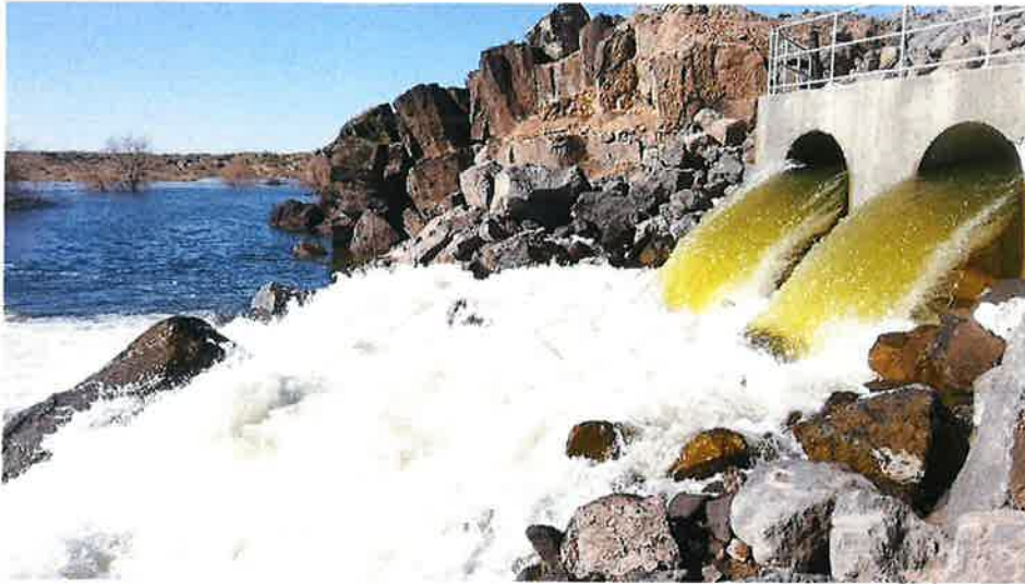
Eastern Snake Plain Aquifer Recharge at the Wilson Canyon Recharge Site
