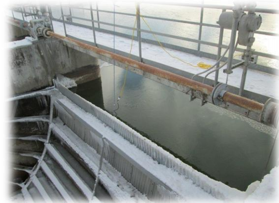
Icing on Murtaugh Lake outlet gates, Nov. 2014
