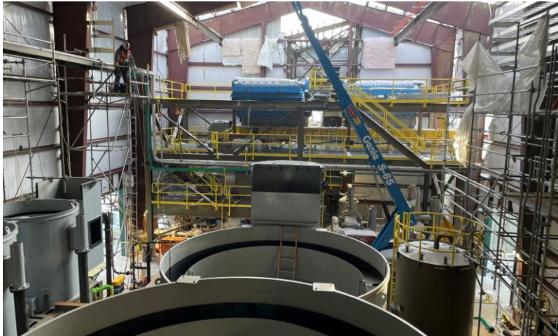
Concentrator progress (January 2023)
