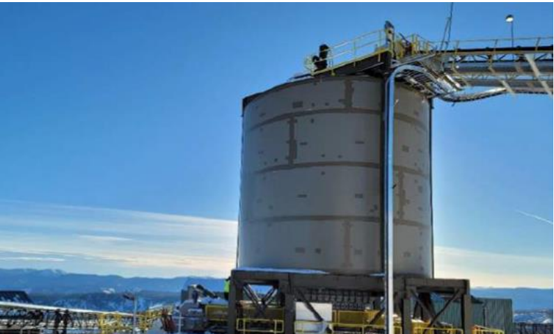
Pre bin area progress (February 2023)
