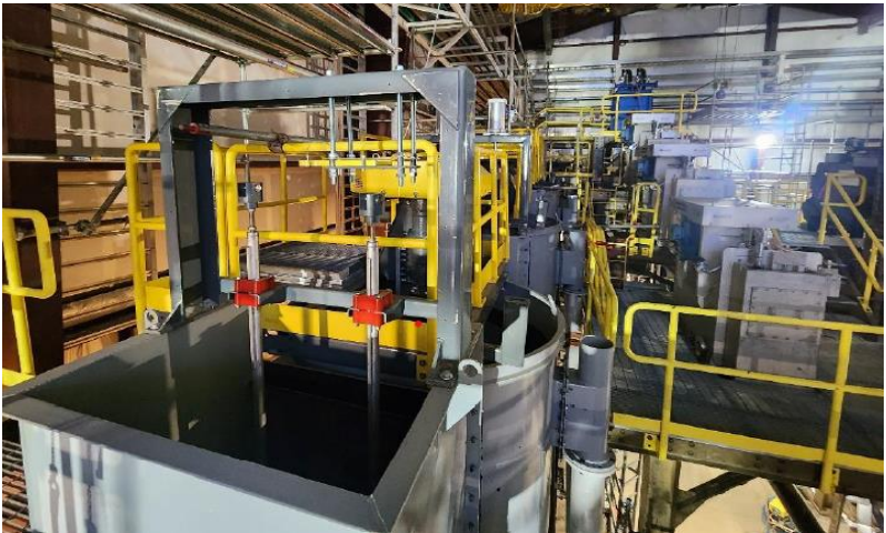
Concentrator progress (January 2023)
