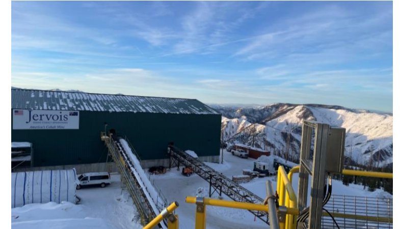
Surface construction (January 2023)
