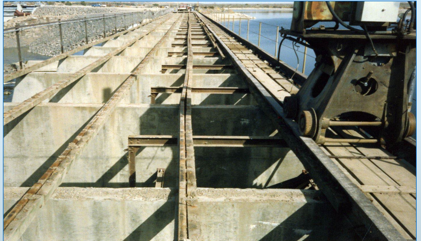
Milner Dam – Spillway Repair
