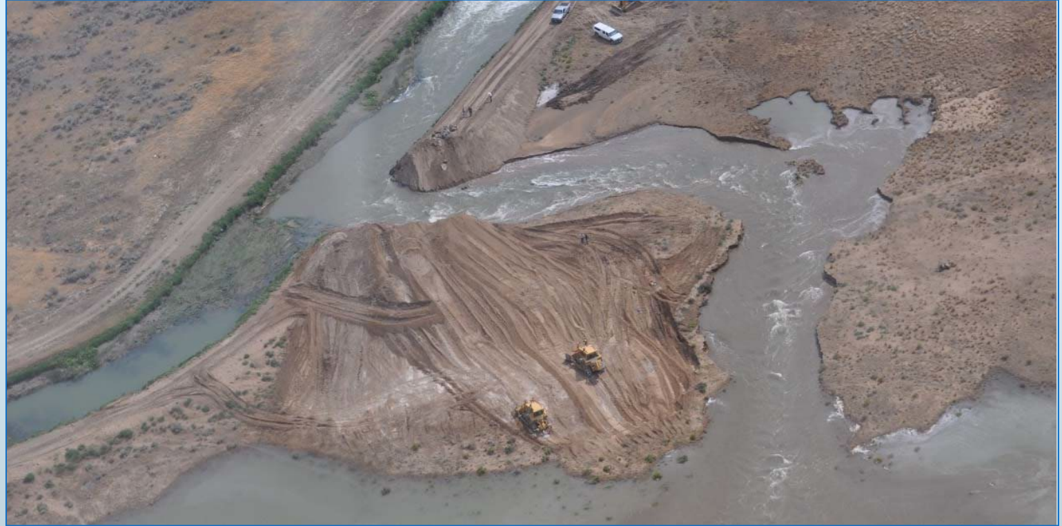
North Side Canal Flood Repairs
