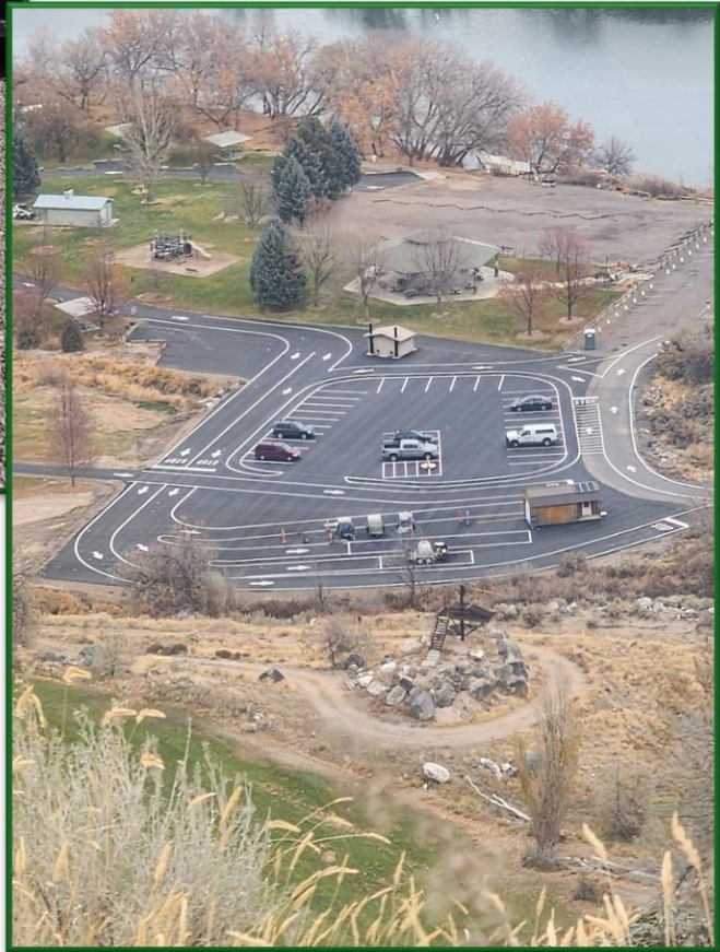
Pavement and Striping
