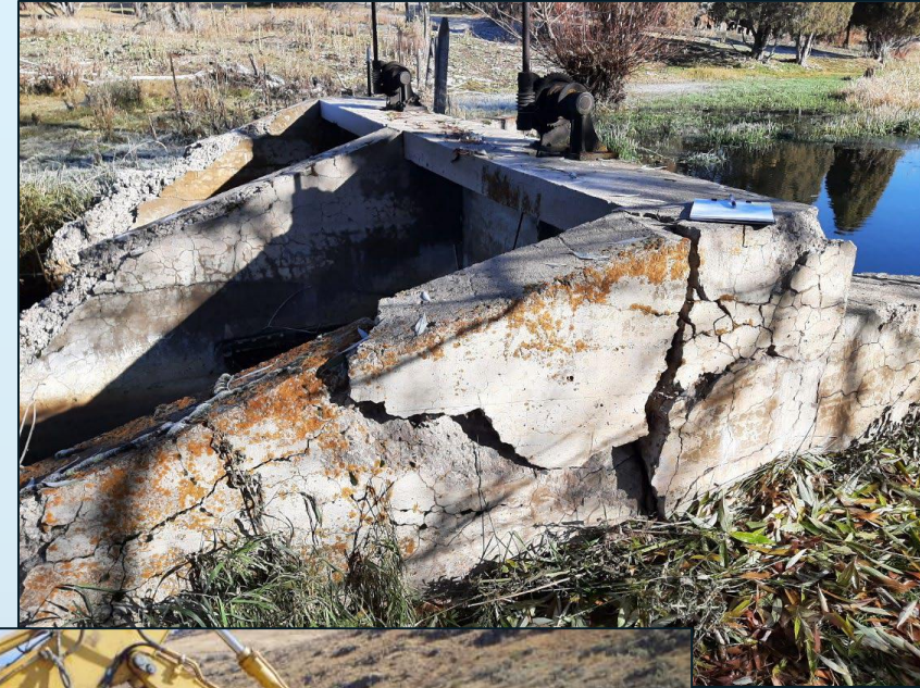
Farmers Land & Irrigation Co. – Soda Creek Diversion Repairs
