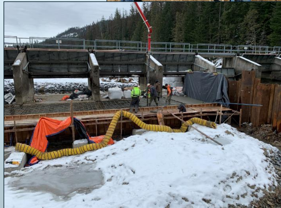
Priest Lake Outlet Dam Modification Project (COMPLETE)
