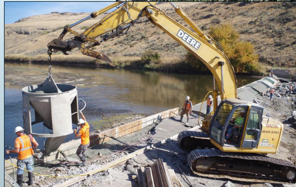
Galloway Diversion Dam Rehabilitation Project
