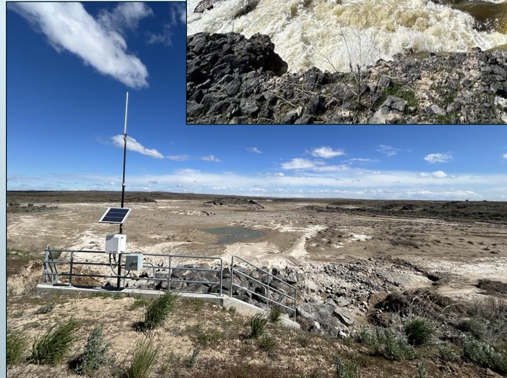
Wilson Canyon Recharge Site Telemetry Installation
