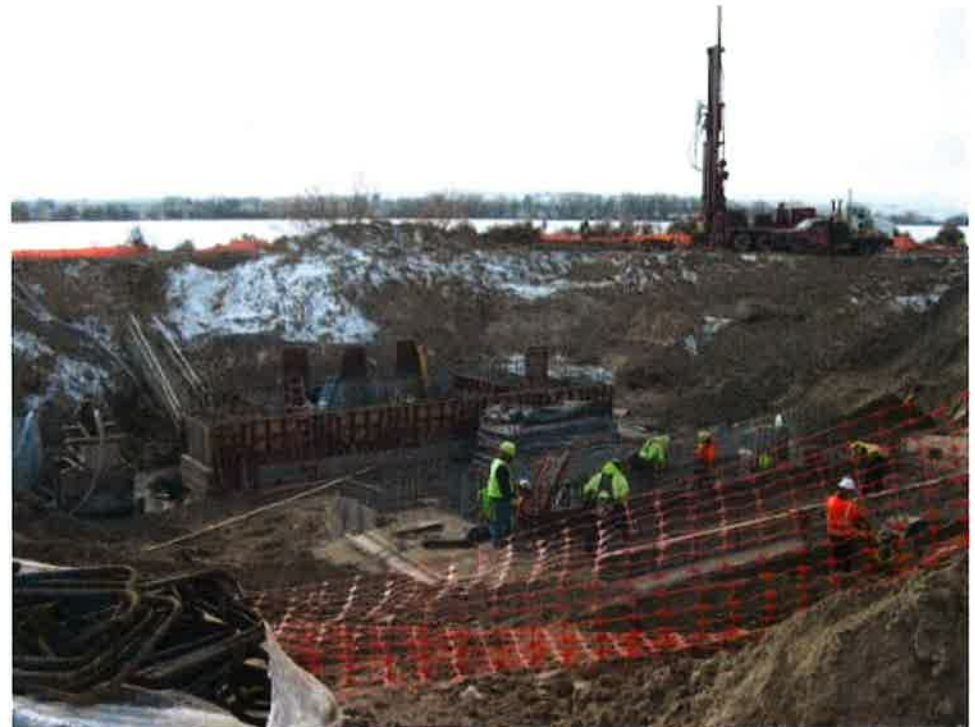
New pump station under construction at A&B Irrigation District, January 2016
